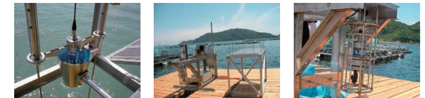
■ Raft-mounted winch system
